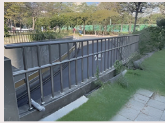
不鏽鋼欄杆已修復完成 Stainless steel railings have been repaired
