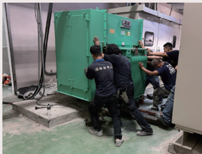
南館變電站更新 South Complex Substation Updates
