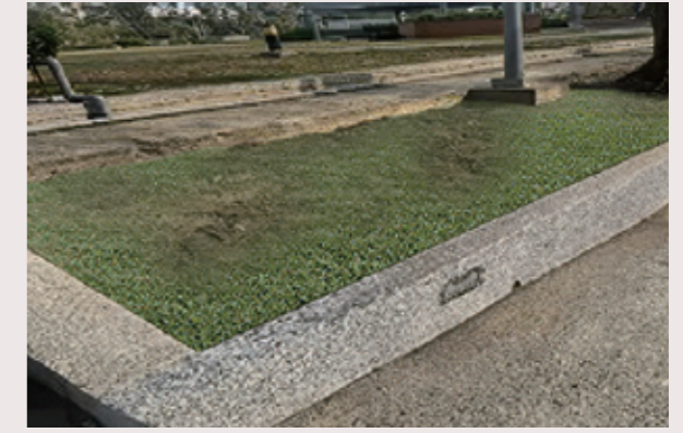
植栽矮擋牆已修復完成 Planting low walls have been repaired
