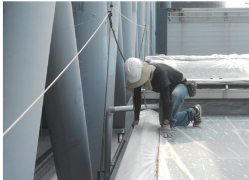
Skylight leakproof canvas replacement operation
