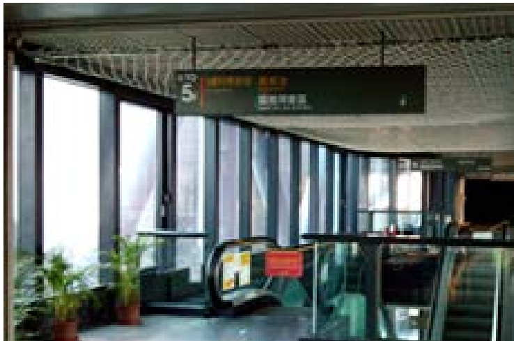
The safety net attached to the ceiling above the escalator
