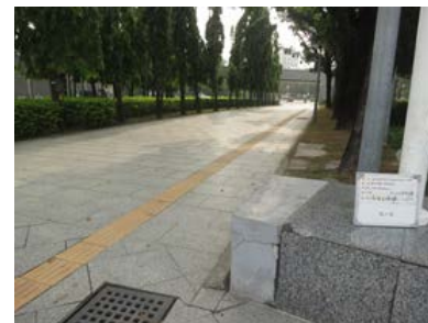
G. Filling of existing outdoor flooring gaps: the filling material was washed away by rainwater and the marble flooring became loose as a result. The gaps were filled again to fix the marble.
