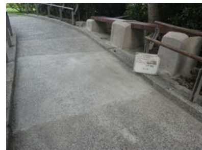
D. Improvement of scrubbed pebble finish: improved the broken access ramp and the appearance of the museum
