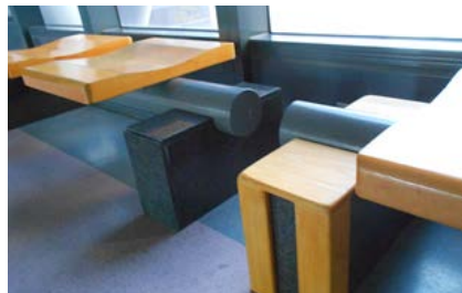
The acute angles of the stone-wood row seats improved with wooden covers
