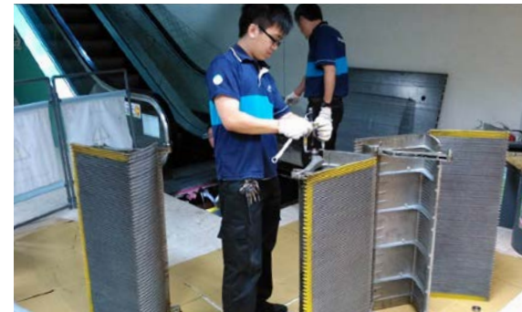
Inspection and replacement of escalator step wheels
